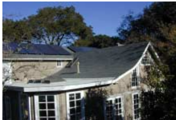
2.0 kW AC Grid-connected, net metered
