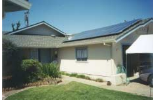
1.6 kW AC Grid-connected, net metered, battery back-up
