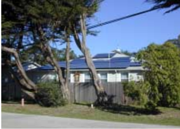
9.0 kW AC Grid-connected, net metered, battery back-up
