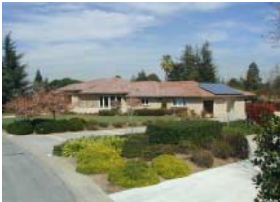
6.2 kW AC Grid-connected, net metered
