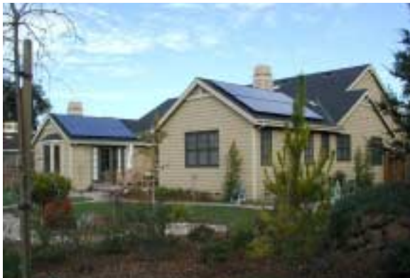
4.0 kW AC Grid-connected, net metered, battery back-up
